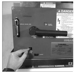
Fig. 27 Manually Opening Breaker
